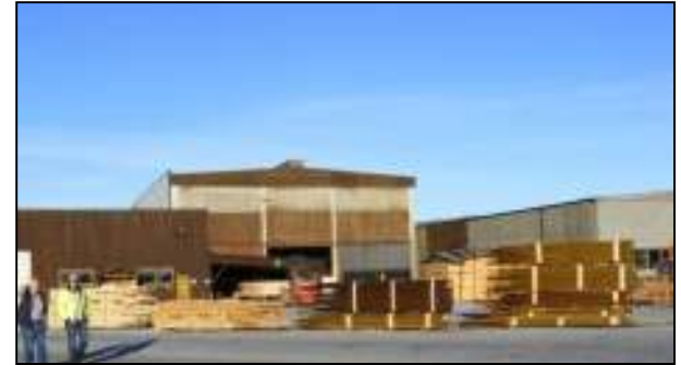
More –Tre plant facility
