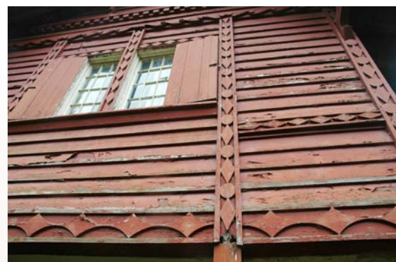
Figure 15: The post at the bottom of this image has been replaced
