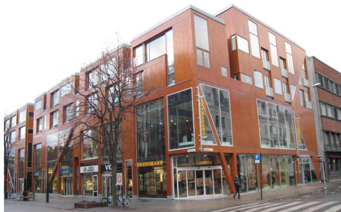
Laminated timber used in a modern trade centre in Trondheim; photo: editor
