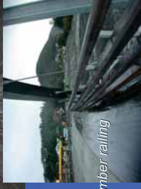
Stress laminated timber deck
