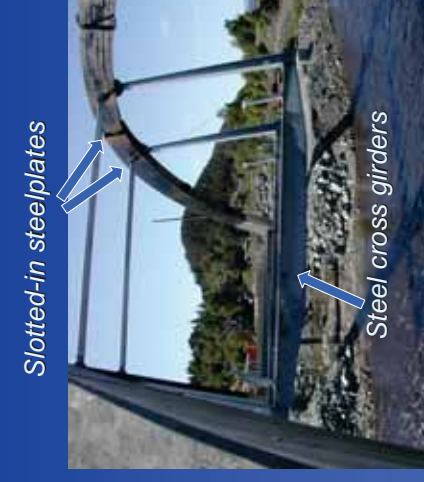
Stress laminated timber deck
